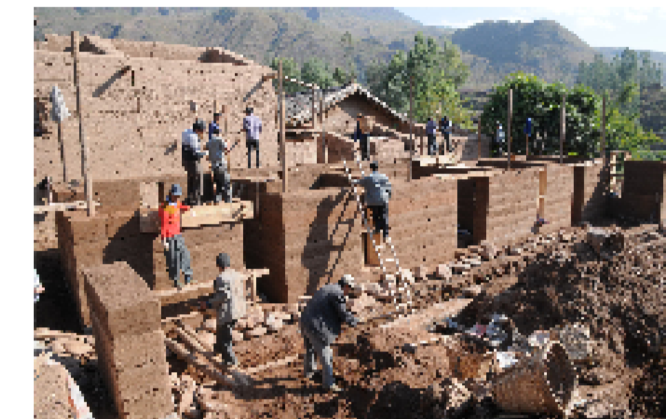
Figure 6. Prototype house construction
