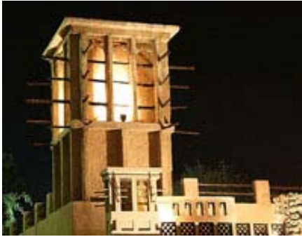
Fig.1 Vernacular materials is used in wind-catchers
