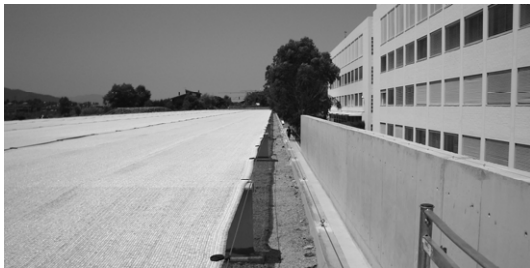
Fig 8. White mesh installed on the roof
