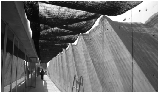
Fig 9. Black mesh installed over exterior corridor on the north façade
