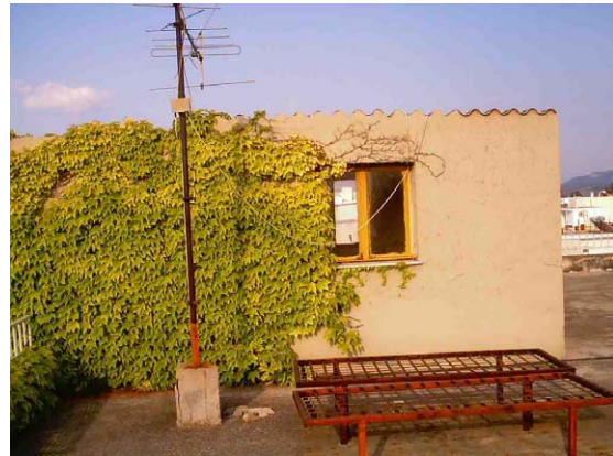
Fig 1. Photograph of the west wall of the room.
