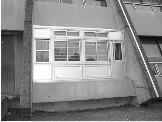
Fig 1. Hybcell test cell facade
