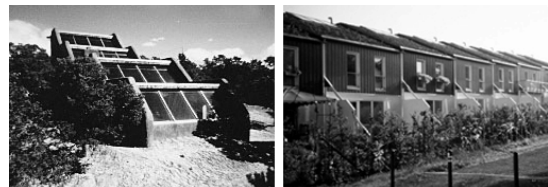
Fig. 04: Karen Terry House and Hannover Passive Houses (Source: Feist, 2003)
