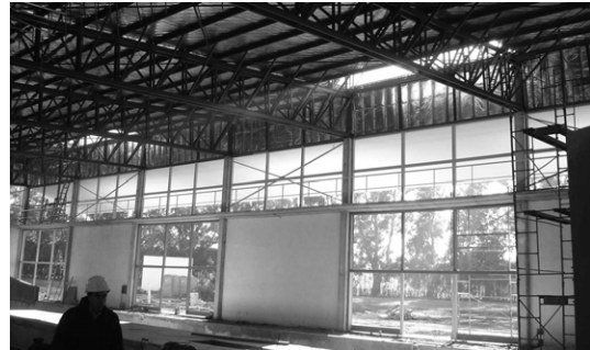
Fig 11: Water therapies building under construction. NE façade and skylights.
