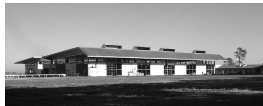
Fig 2: Water therapies building. NE view.
