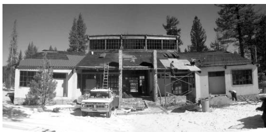
Fig 1. Southern view of the site (under construction in February 2008)
