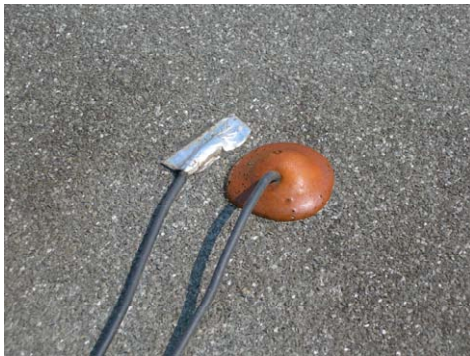
Fig 1. T1 and T2 probes on the roof
