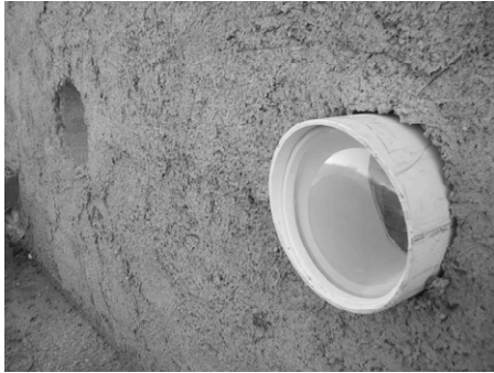
Image 6. Window made of a sewer pipe and a dinner plate set in papercrete wall.
