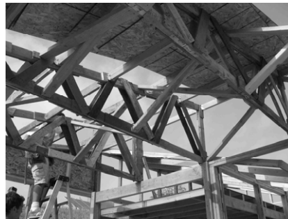
Image 5. Wood pallet roof truss system
