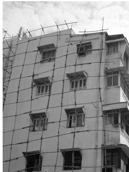
Fig 2. Bamboo scaffoldings in Mumbai (India).
