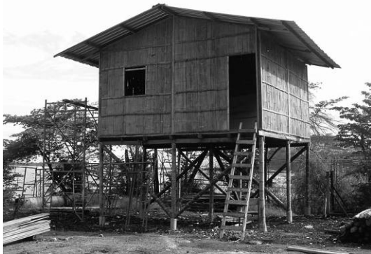
Fig 6. Prototype of a house designed and realized by the architects Gabriele Casu and Giuseppe De Nunzio in Guayaquil (Ecuador) for the Organization Hogar the Cristo. (image by Casu and De Nunzio)
