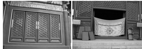
Fig 6. Windows and door with lattice
