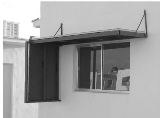
Figure 6. Solar protection device added to the windows.
