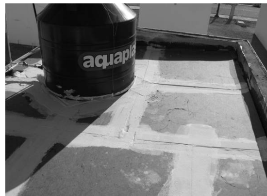
Figure 7. Additional insulation applied to the roof.
