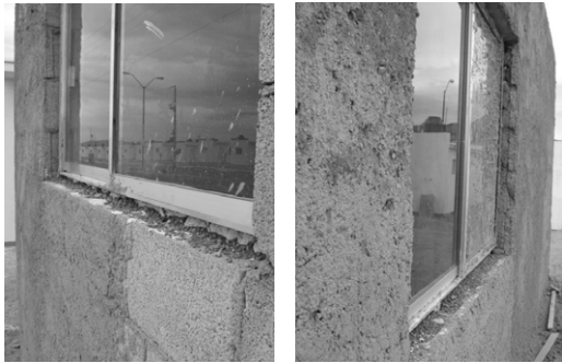
Figure 8. Concrete blocks filled with earth
