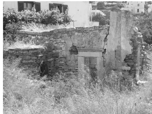
Fig 7. Façade of abandoned traditional house with channel for rainwater.
