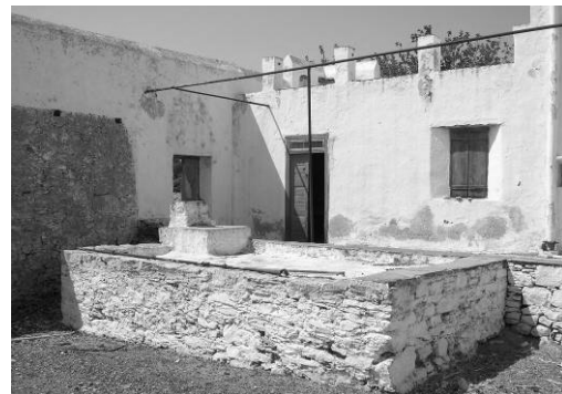
Fig 14. Cistern in the centre of the yard of a country-house (Mousia) on the south of the island.
