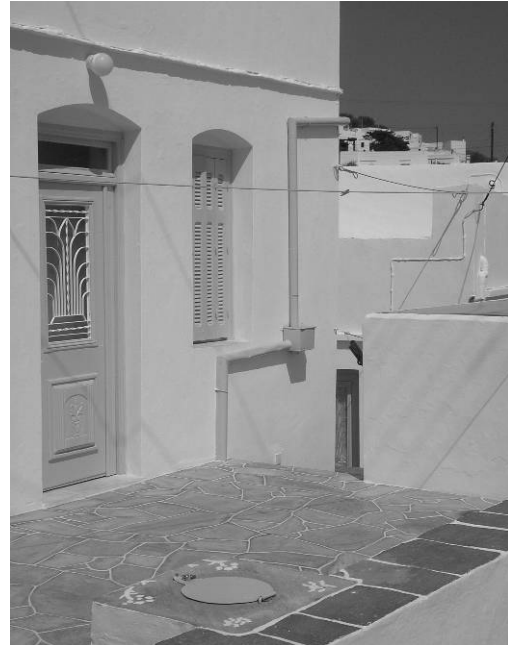
Fig 13. Cistern below the front yard of a house in Artemonas, with gutter with the tin box and well-like opening.
