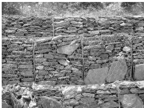
Fig 20. Slate rocks in prefabricated steel frames.
