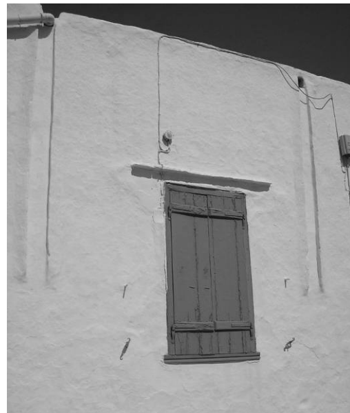
Fig 8. Façade of traditional house with two channels for rainwater.
