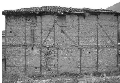
Fig 17. House in Florina built with the local structural system
