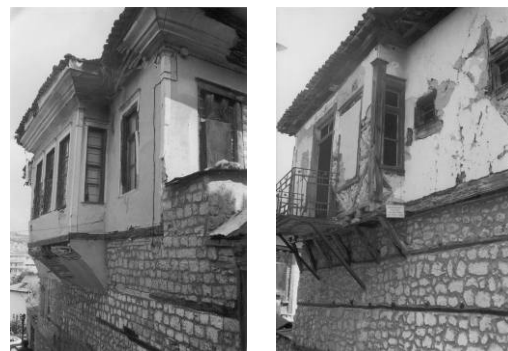
Fig 18. Houses in Veroia built with local porous stone and lightweight timber frame walls
