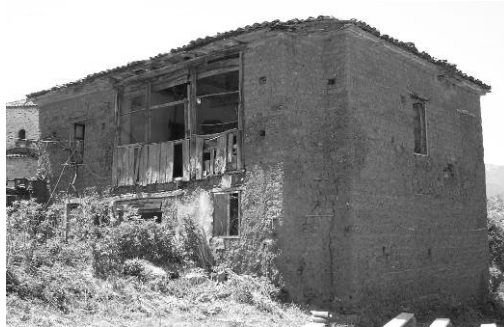
Fig 14. House in Ano Kranionas built with adobe
