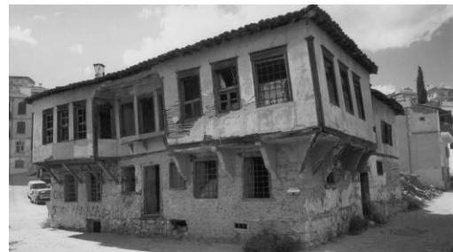
Fig 11. 19 th century house in Kastoria
