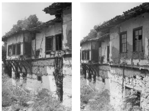
Fig 15. House in Eratyra built with stone and lightweight timber frame walls filled with fired clay bricks
