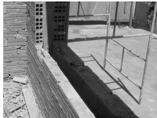
Fig 6. Double brick walls with cavity
