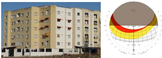
Figure 7. bad designs and bad shading masks, cause glare, summer overheat and winter heat lose.
