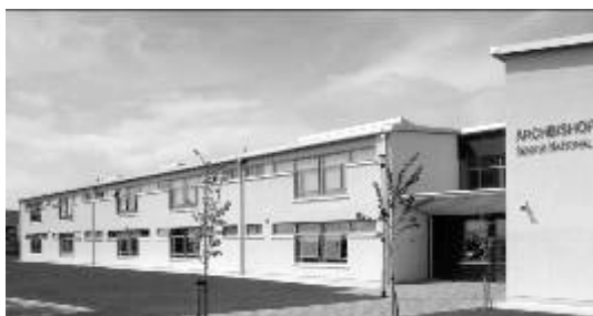
Fig. 1 South facing 2-storey classroom block & entrance of first completed GRD School.
