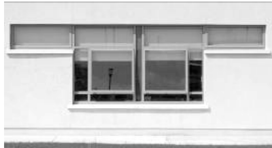
Fig 11. Typical Classroom windows.
