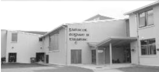
Fig 8. North Entrance with canopy.
