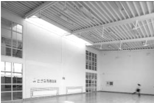
Fig 13. School Hall – balanced glare-free daylight from windows and high level roof lantern.
