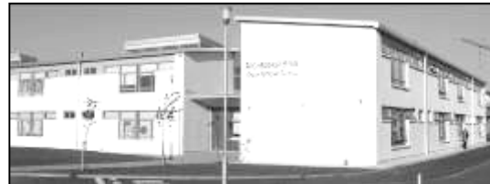
Fig 15. South & East facing classroom blocks with South Entrance between.
