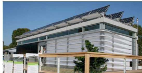
Fig. 1. Southeast Corner, Georgia Tech Solar Decathlon House, 2007
