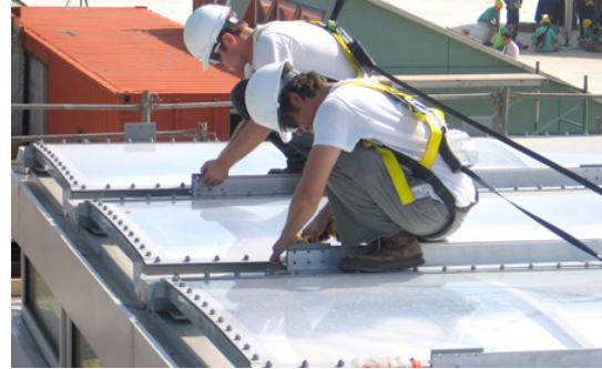
Fig. 5. Translucent Double-Skin Roof, Georgia Tech Solar Decathlon House, 2007
