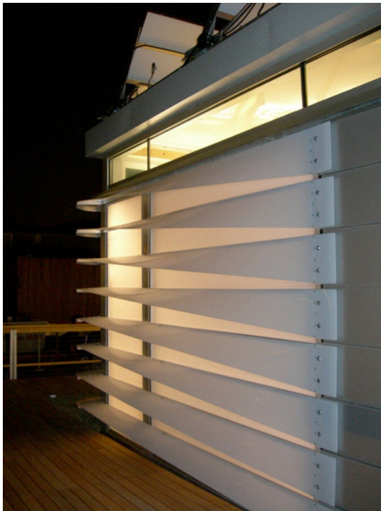
Fig. 7. Polycarbonate Screen, East Wall, Georgia Tech Solar Decathlon House, 2007
