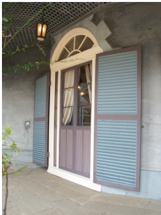
Fig 7. French window with movable louver open to the verandah.
