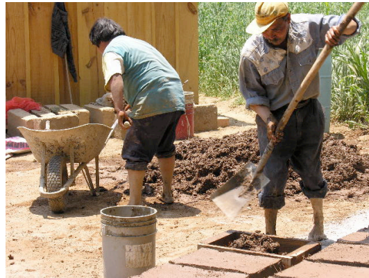
Fig. 2. Local builders preparing the adobe
