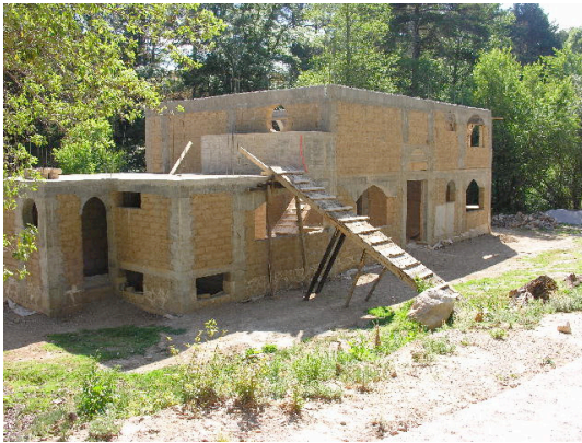
Figure 1. Overview of Case Study Building
