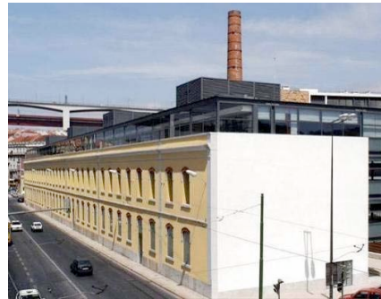
Figure 4 – Refurbishment of the "Union" factory, into housing and commerce, in Alcântara, Lisbon
