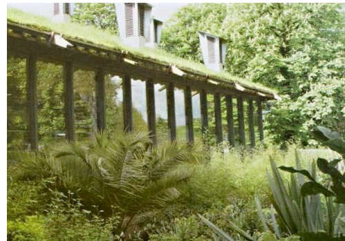
Figure 8 – Green Roof in "Centre for Understanding the Environment", (Source: Harrington, 2005)
