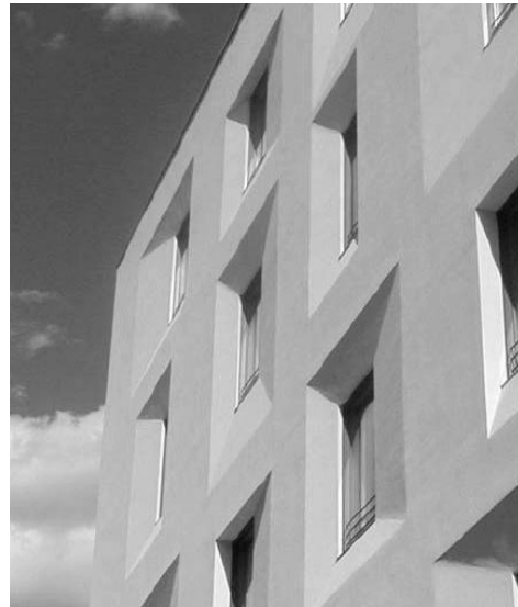
Fig 4. Detail of realised Façade
