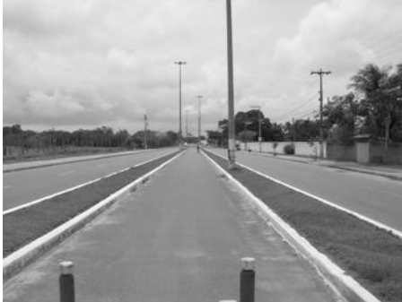
Fig. 6 - Main way with bicycle paths, but without no protection against the direct solar radiation.
