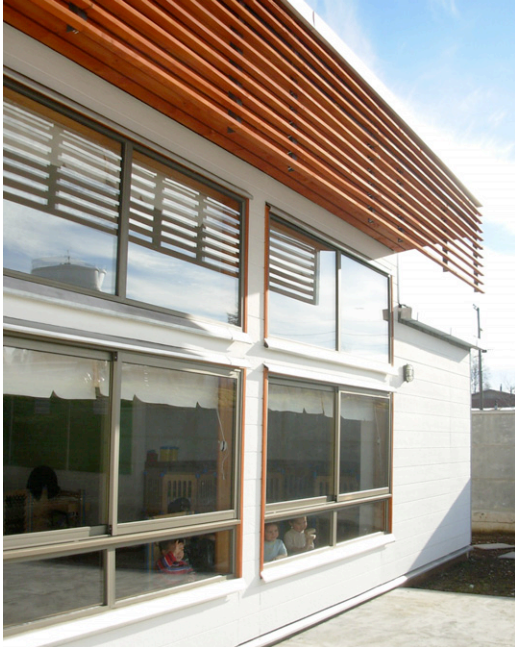
Fig 6. Nursery school of Villarrica. Chile.
