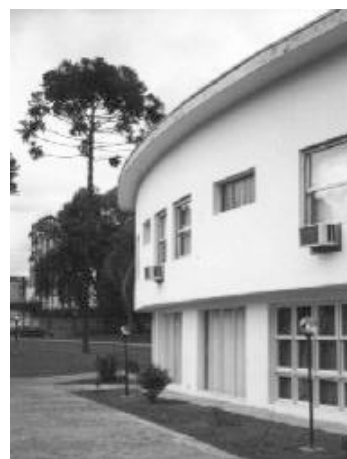
Fig 7. Northwest curved façade [4]
