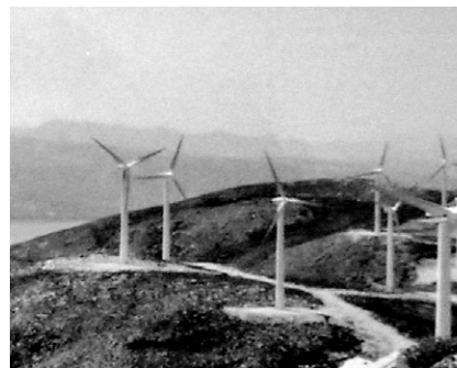
Fig 5. Photo of Wind Farm [3] (Euboea Island)
