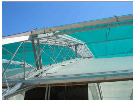
Fig 2. Detail of the roof, the truss structure and the upper and lower foil
