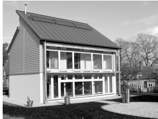
Fig 5. View of BASF House from the South (Source: BASF [6])
