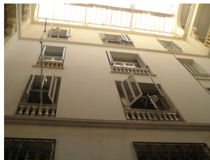
Picture 3: Upward view of the atrium, south east façade, autumn campaign 2006
