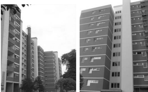
Fig 2. The Austrian Demonstration building, before (left) and after renovation (right).
