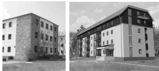
Fig 5. The Hungarian Demonstration building before renovation (left) and artist impression of post-renovation state, showing the rooftop apartments (right).
