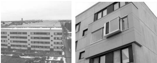
Fig 3. The Danish demonstration building, before renovation (left). On the right a single test apartment with external insulation.
