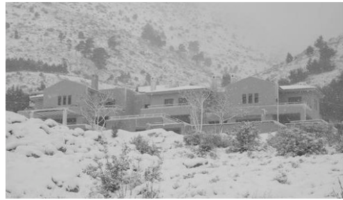
Fig 4. The Greek Demonstration building, during construction and after completion. The picture above shows that weather conditions can be severe and good thermal insulation will pay off.
