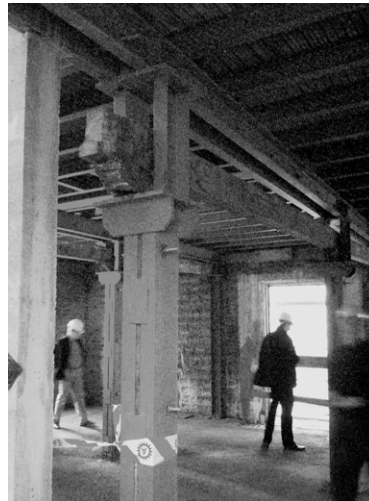
Fig 6. Structural reinforcements were necessary in the Spanish project.
