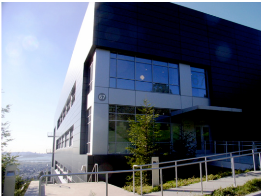
Fig 5. Berkeley Lab's Molecular Foundry –East and South Elevations
