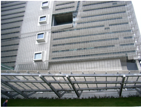
Fig 9. The San Francisco Federal Building – South Elevation with perforated metal skin as horizontal Sunshades
