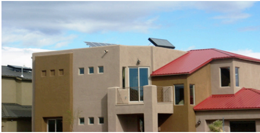
Fig. 13. Hose in Civano II –PV Panel and Solar collector for hot water. No Passive Solar Architecture.
