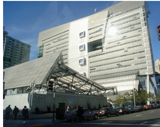
Fig 7. The San Francisco Federal Building – South Elevation and the restaurant in the front of it
