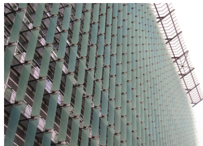
Fig 8. The San Francisco Federal Building – North Elevation with vertical glass fins as brises-soleils
