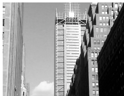
Fig 1. The NYTB during final construction phase. Feb 2007
