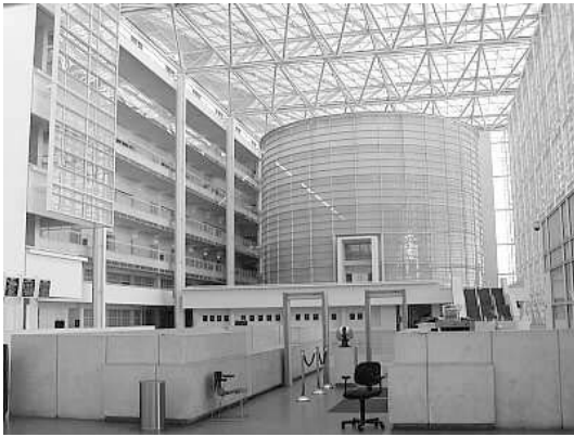
Fig 1. Building 1 - Sandra Day O'Connor Federal Courthouse, Phoenix, AZ
