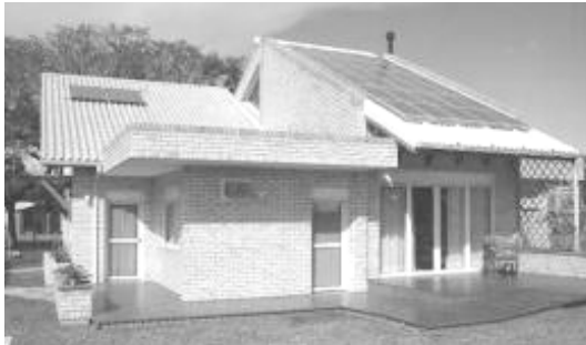
Fig 2. North façade of the Efficient House
