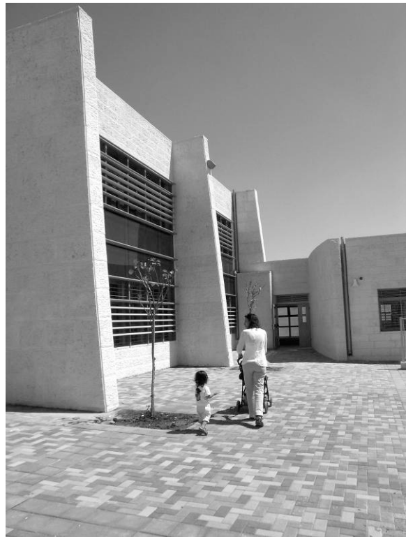
Fig 7. View from south
