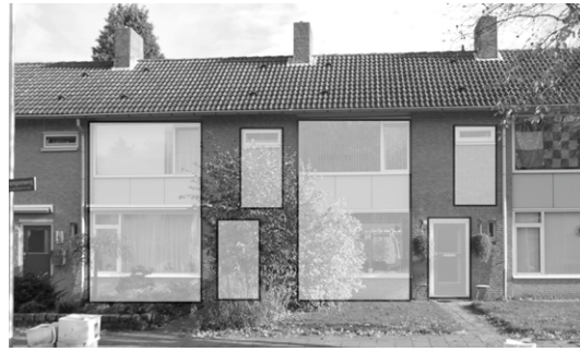
Fig 2. Configuration of the façade. The openings that will be created are shaded.
