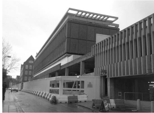
Fig 2. Existing east block before the removal of the existing cladding panels
