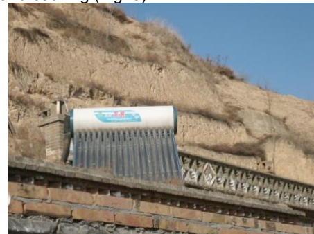
Fig 5 Solar thermal technology for water heating (picture taken by YAO Jiali in the Gaoxigou Village, Shanbei region)
