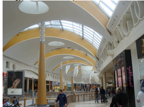
Figure 5 – The roof lights
