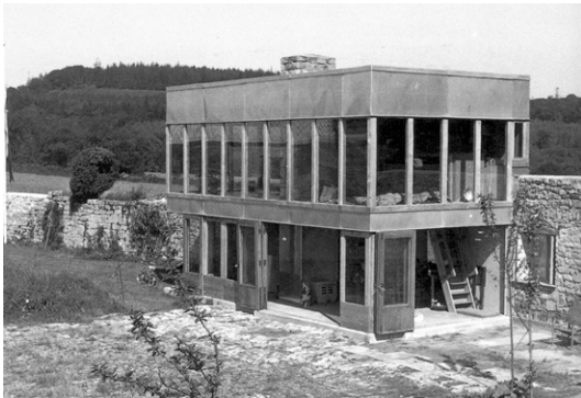
Fig. 9 Upper Lawn, view from south-east
