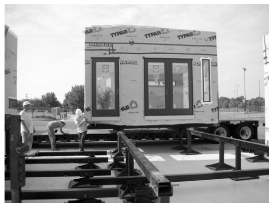
Fig 4. A rail system as temporary foundation and assembly line
