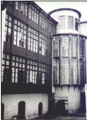
Figure 8: Former Fieschi hotel built in 1858 and restored between 1975 and 1977, Bucharest, Sun Street
