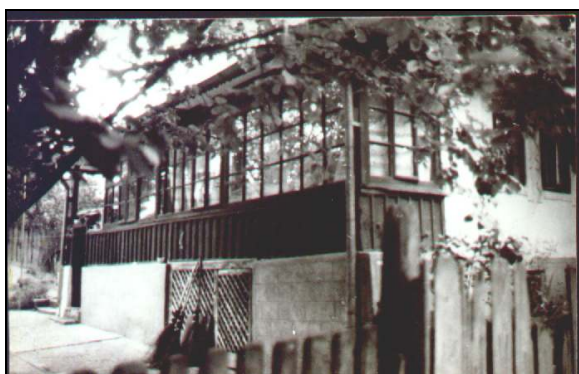
Figure 3: Late 19 th century house with porch closed with glass panels – Campulung town, Muscel County.
