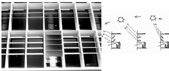
**Figure 2:** Detail of the lumiere and sketch by Lúcio Costa showing the way it works.
