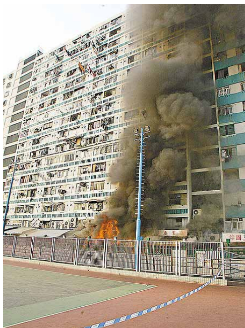
(a) Restaurant fire due to flashover (Apple Daily, 7 January, 2005)
