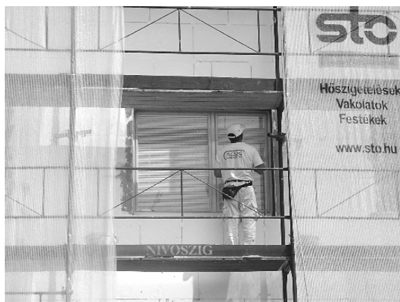
Figure 5: The facades were covered with 16 cm polystyrene thermal insulation
