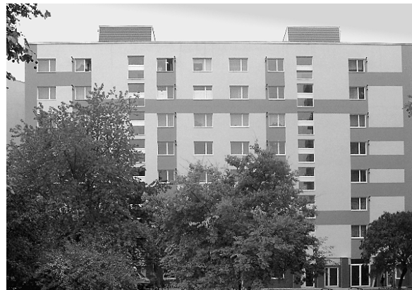
Figure 2 The Solanova building after renovation
