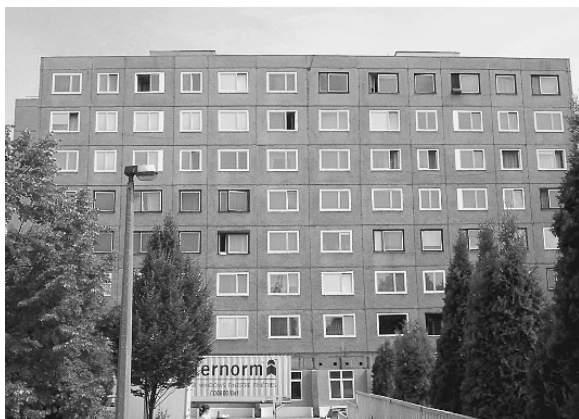
Figure 1: The Solanova building before renovation
