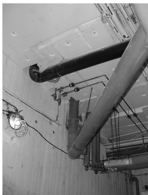
Figure 8: Insulation of cellar ceiling with 10 cm PS
