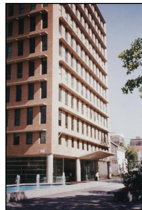
Figure 5: Building Pedro de Valdivia. East oriented entrance.
