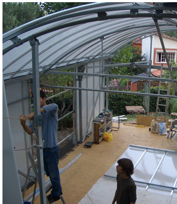
Figure 1: Image of the greenhouse-studio during the building process.
