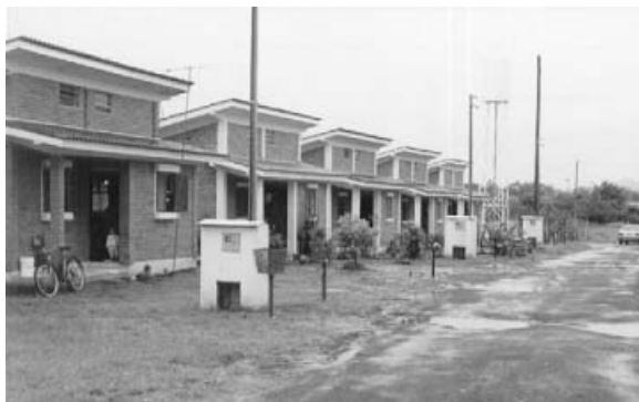
Figure 2: General view of CETHS.
