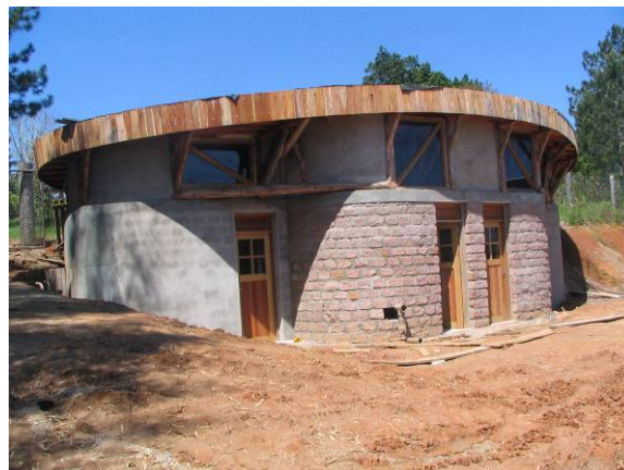
Figure 1: The school building being monitored.
